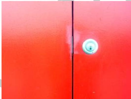
*Lock sets like the one shown here can be easily forced open. In absence of an engineered access control system, latch guards should be installed to lessen the risk of forcible entry.*
