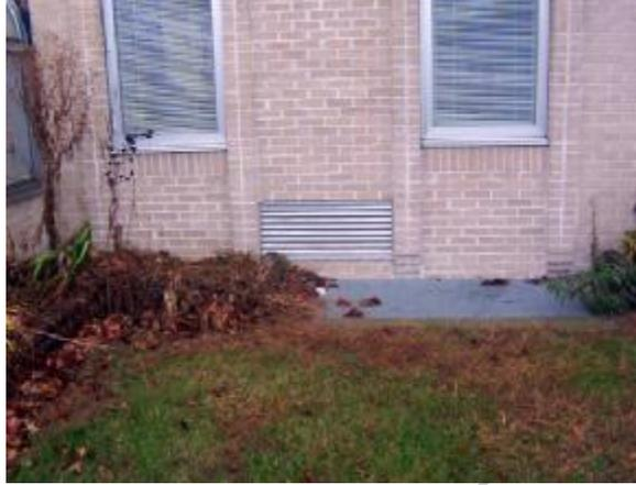
*Once thought of as nearly harmless, air intake louvers must now be considered a risk factor for the introduction of poison or toxic gases into the air handling system, and should be protected accordingly.*
